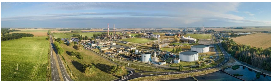
Picture: View of the site in Grandpuits, France where Total Corbion PLA intends to build its second Luminy PLA plant with a capacity ramping up to 100,000 tons per annum.
